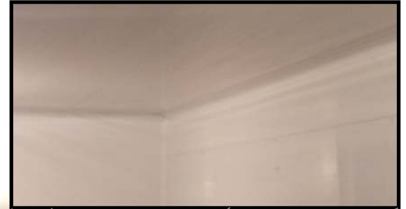
This cooler space was finished with Trusscore PVC panels resulting in a smooth, cleanable surface.
